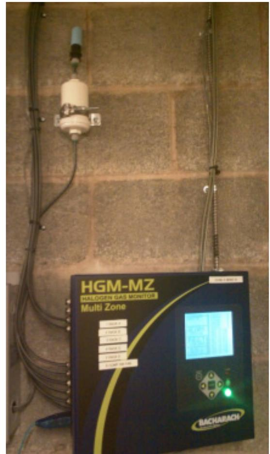
Figure 7. Indoor Filter Mounting Example
